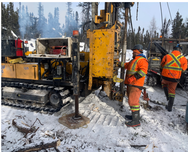
Geotechnical drilling of bedrock for wind tower mounting. Photo owned by SDFN courtesy of Kisik Clean Energy.
